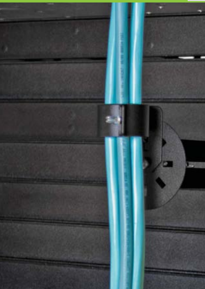
Rack-Mount Universal Clamp Kit Installed
